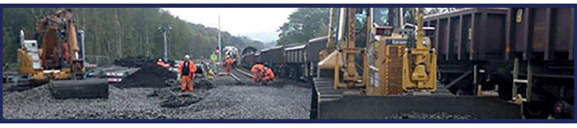
The Todmorden Curve project – to reinstate a 400-metre stretch of rail track, which had been closed since 1972 – was a project completed by Haigh Rail Ltd. The company's services were vital in enabling the first direct service to run between East Lancashire and Manchester in more than 40 years.
