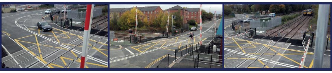
Spondon Level Crossing was a unique job that Haigh Rail recently undertook on behalf of partner Siemens Rail Automation. The works consisted of a full level crossing deck renewal, plus realignment of the existing footprint to accommodate a new alignment of the highway.
