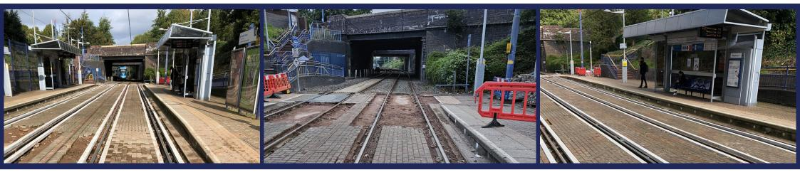
Haigh Rail Limited were tasked with concrete remedial works, baseplate re-alignment, re-railing, crossing replacements, block paving replacement and re-gauging of all four corners into the stops at two locations, Dudley Street and Dartmouth Street tram stops.
